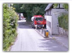
Road narrowing simply reduces the width of the road. This could be achieved in several ways, however a technique commonly used extends the curb into the road at a junction entrance with a bollard on each side.
