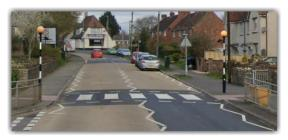
Zebra crossings help pedestrians cross from one side of the road to the other. They have white strips painted onto the road in the crossing area, with flashing amber lights at both sides of the road on black and white striped poles. The curbs are dropped at both ends of the crossing, usually with tactile paving where the pavement slopes towards the road. Vehicle users can see zigzag lines on the approach to the crossing, sometimes with a buff-coloured road surface.
