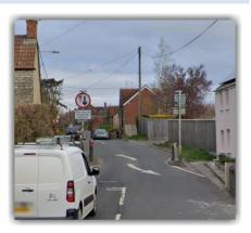
Groups of chicanes are normally placed with alternating priority down a road, so that each direction of vehicle traffic may have to stop and give priority in equal amounts.
