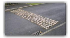
Rumble devices are small, raised areas across the carriageway with a vibratory, audible and visual effect. They are used, usually in rural areas, to alert drivers to take greater care in advance of a hazard such as a bend or junction. In combination with a gateway, they can indicate the entry to a village or the start of a series of traffic calming measures. They have also been used to designate the start of shared use roads in new developments.
