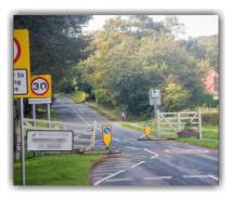
The village gateway helps to create 'a sense of place' when drivers enter the village, and the physical measures are designed such that drivers are required to slow down before entry.
