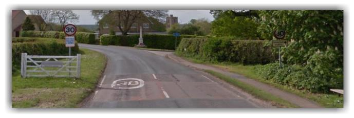
These gateways only have signs and lines, and always display the village name to introduce drivers to the village. In addition, road markings are used to create a visual impact when drivers enter the village. These markings could be:
